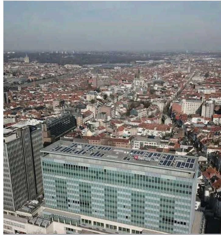
201KW Brussels, Belgium
